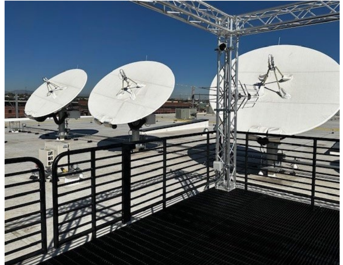
Satellite receiving dishes on the rooftop of Scripps' KMGH/Denver7.
